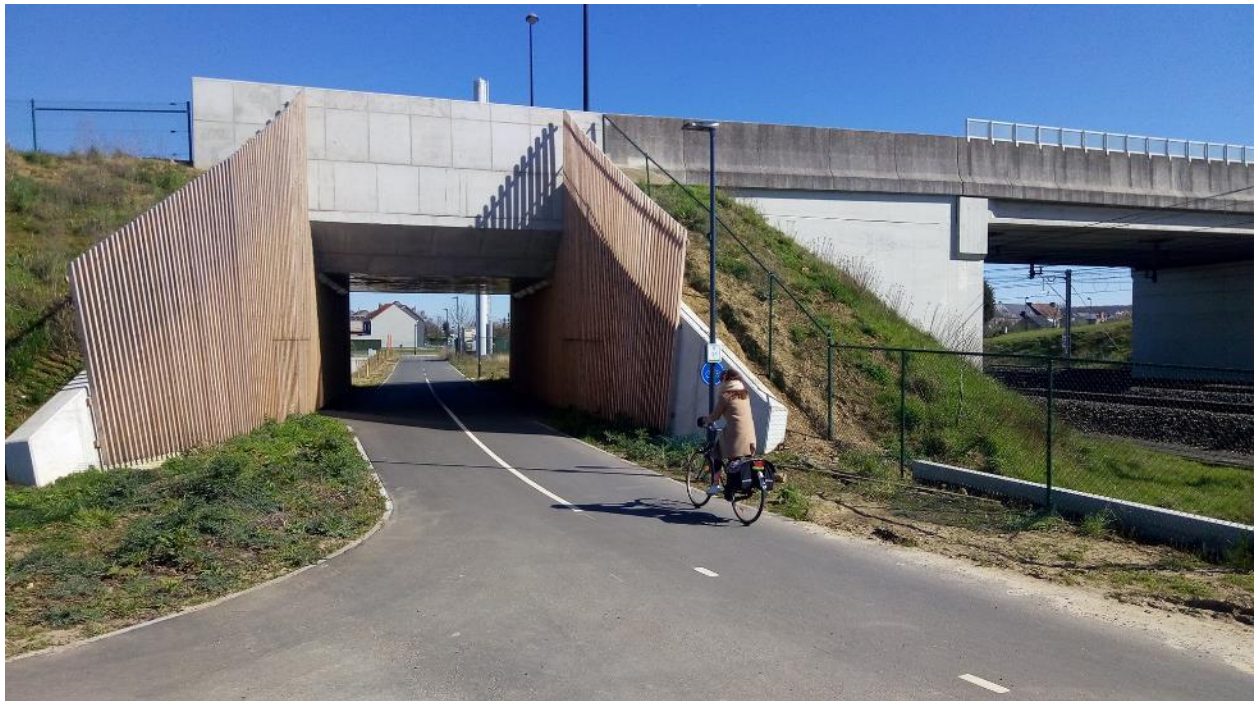
Figure 2. Following railway lines reduces the number of crossings and makes it easier to provide grade separation on them. Cycle highway F3 Brussels – Leuven, Belgium.
