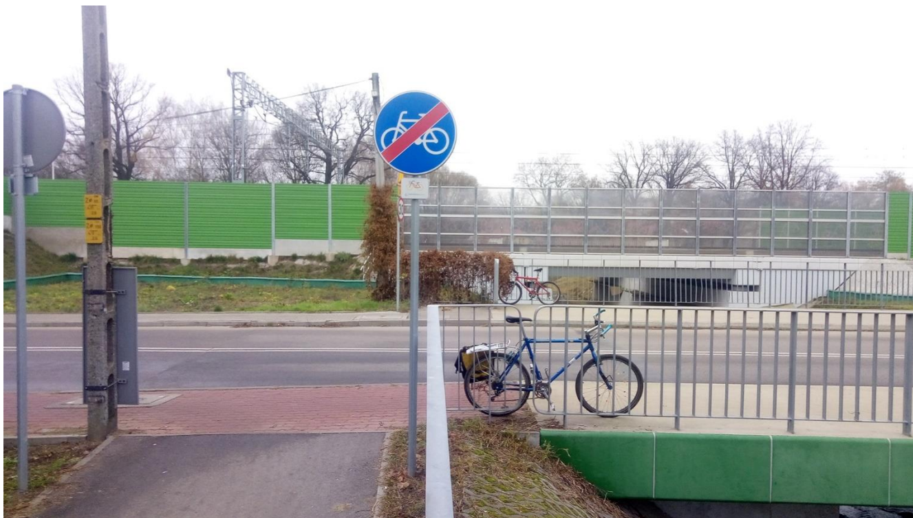
Figure 1. Example of a barrier created by a TEN-T project. A cycle track in the town of Zielonka, Poland (co-funded by the EU through Integrated Territorial Investments) is interrupted by an upgraded section of Rail Baltica (co-funded by the EU through Cohesion Funds).
