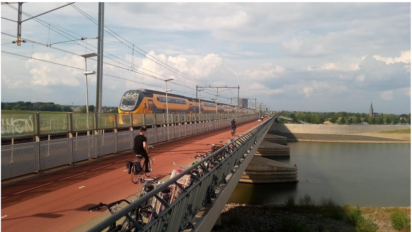
Figure 6. 6,000 cyclists per day use “Snelbinder”, a 2-km long cycling bridge attached to the railroad bridge over the Waal river and embankment in Nijmegen, Netherlands.
