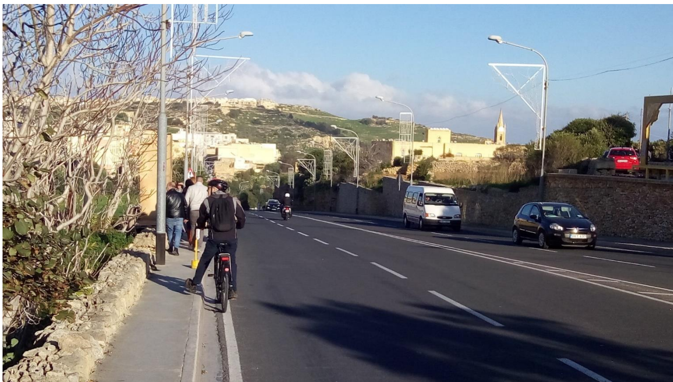
Figure 4. Triq l-Imġarr leads to the ferry between Gozo and Malta, and is an example of a TEN-T road where different modes of transport are mixed. "Upgrading" these roads to serve only motorised traffic needs to be accompanied by providing segregated infrastructure or alternative routes for active modes.
