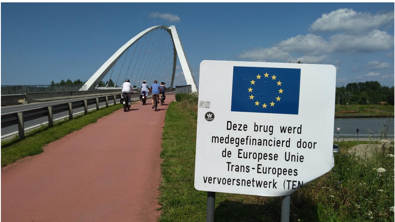
Figure 3. The main objective of the project was to raise the clearance under bridges on Albert Canal (TEN-T inland waterway) in Belgium, but it has also been used as an opportunity to add or improve cycle infrastructure on the bridges.
