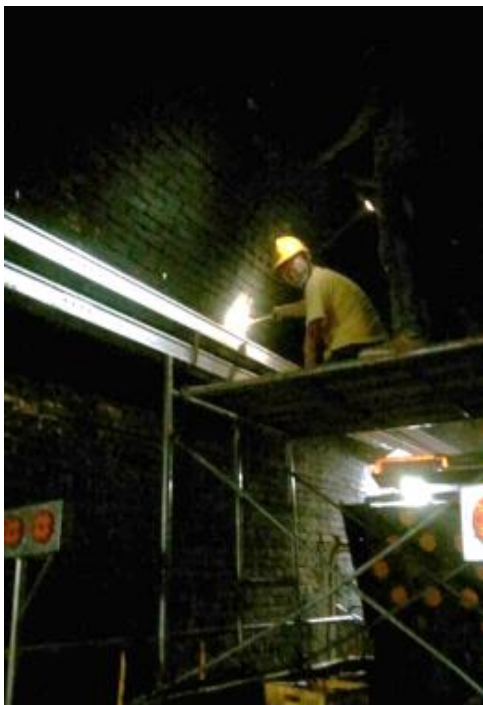
Old Caoling Tunnel Structural Reinforcement Process - Implementation of Safety Netting
