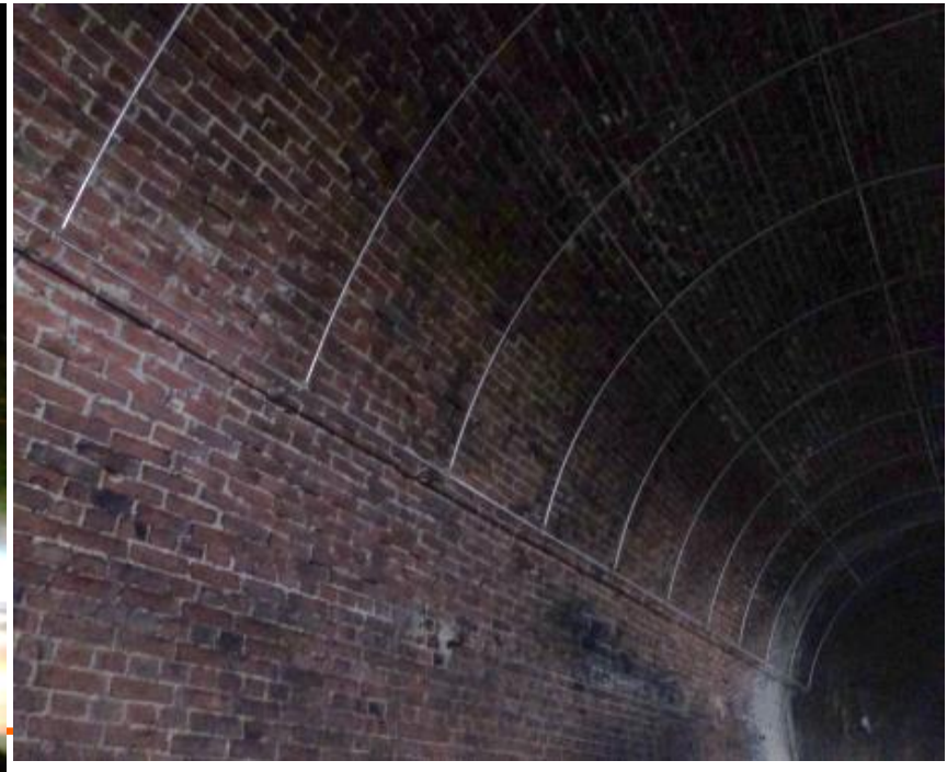
Old Caoling Tunnel Structural Reinforcement Process - Implementation of Safety Netting
