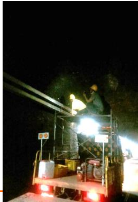
Old Caoling Tunnel Structural Reinforcement Process - Implementation of Safety Netting
