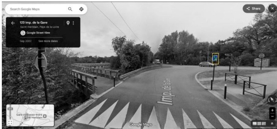
Figure 18 - Access point to the cycling-pedestrian route. The highlighted sign indicates it is accessible to both pedestrians and cyclists. [(3_1)street2_2022]
