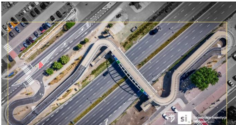
Figure 19 - Aerial view of the bridge showing separate access points and infrastructure leading to and from the pedestrian-cycle bridge. [(3_2)img4]
