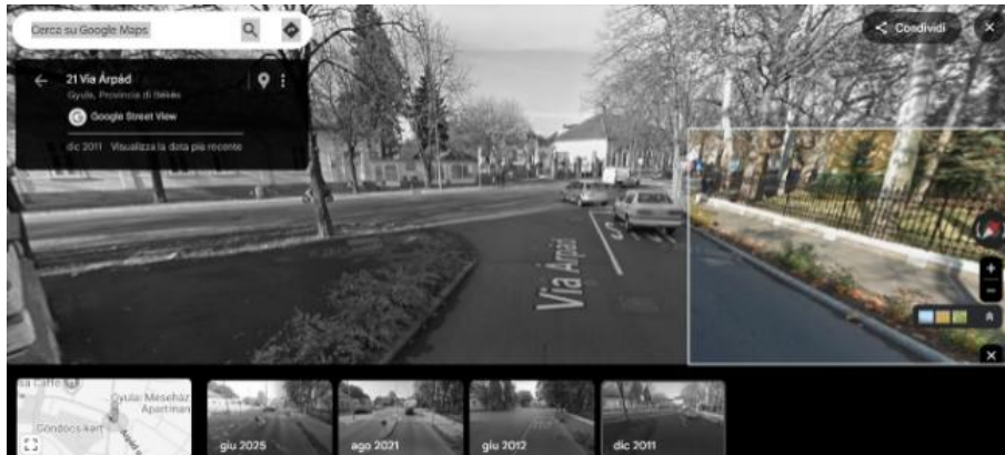
Figure 11 - Street view of Árpád Street showing the presence of sidewalks prior to the development. [(1_2)street_2011]
