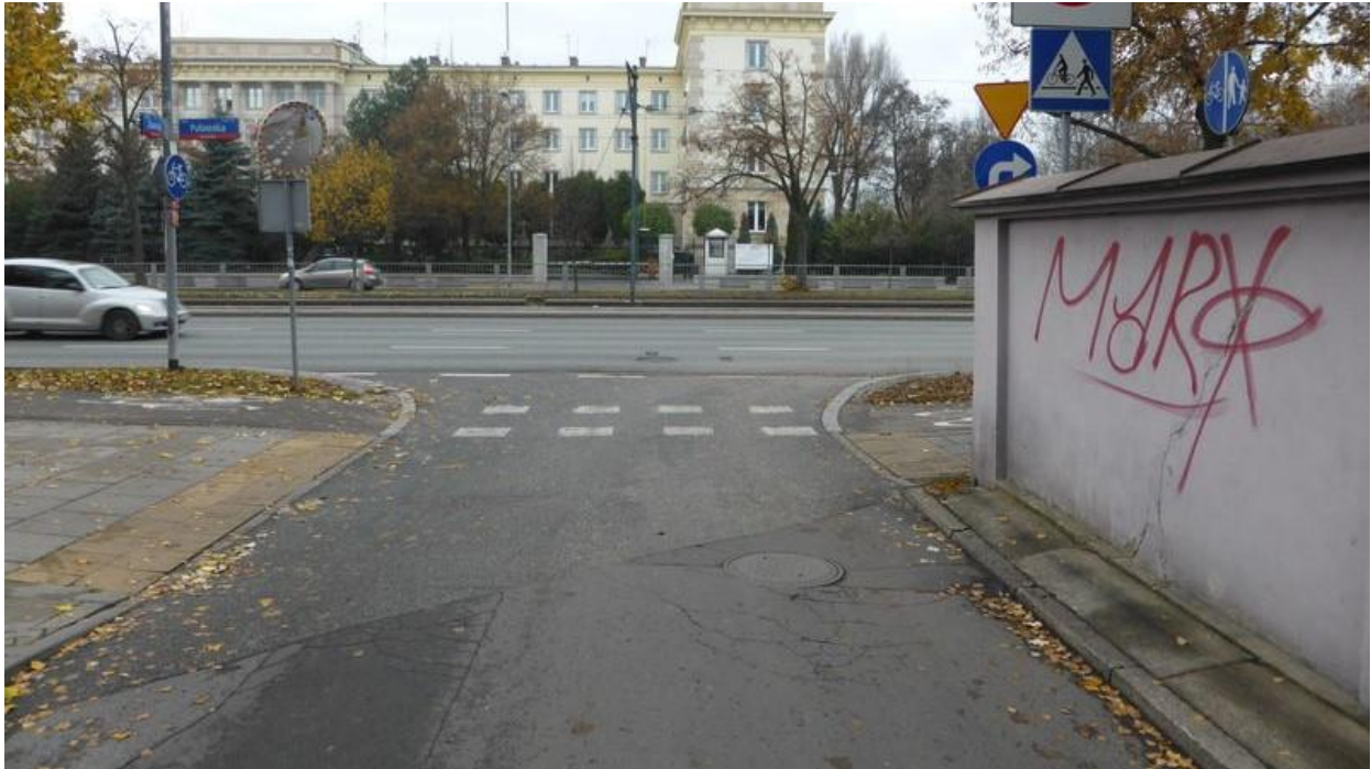
Figure 6. Insufficient visibility splay was a contributing factor in several crashes on the crossing. The problem was remedied by making the street one-way, with contraflow cycling allowed. Warsaw, Poland.
