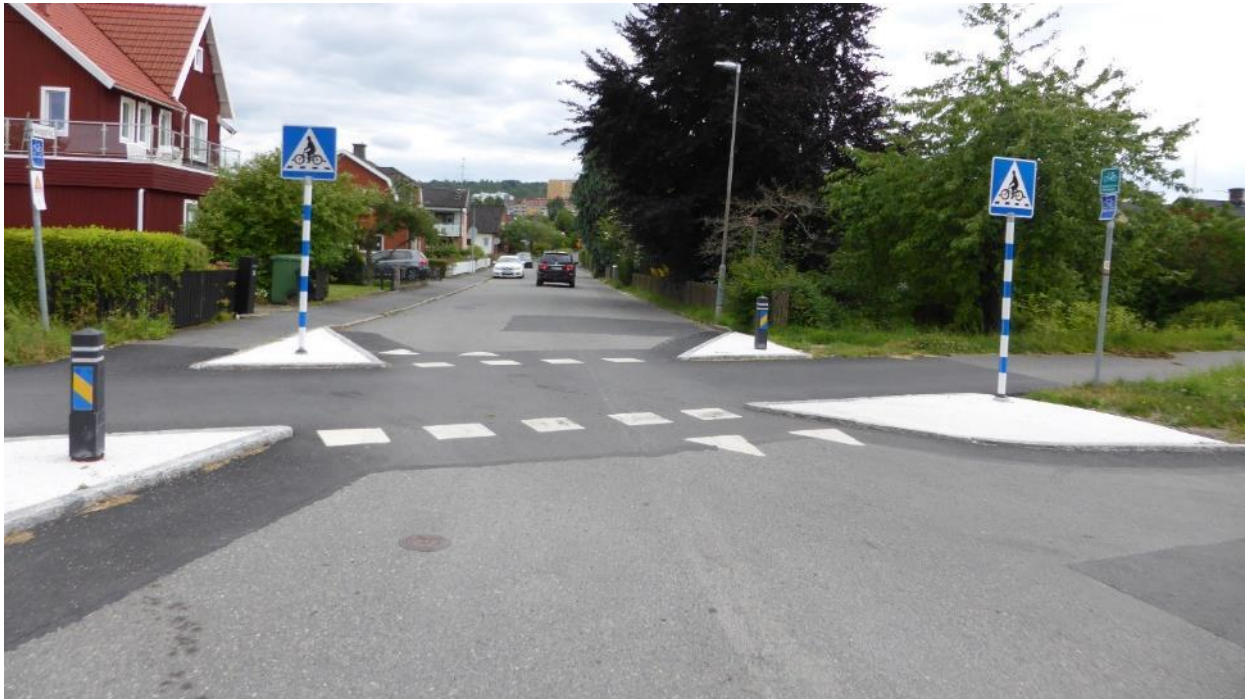
Figure 3. Reduction of the crossing length to improve safety. Jönköping, Sweden.
