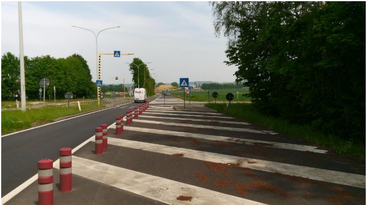
Figure 2. N25 road was reduced to a single lane per direction when approaching the at-grade cycle crossing. Oud-Heverlee, Belgium.
