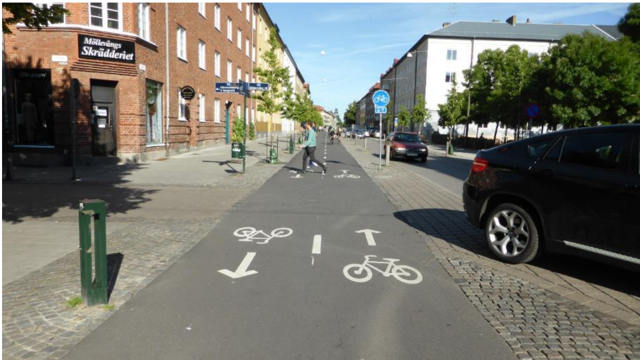
Figure 8. So-called exit from a residential street, with continuity of cycle track across the minor arm of an intersection. Malmö, Sweden.
