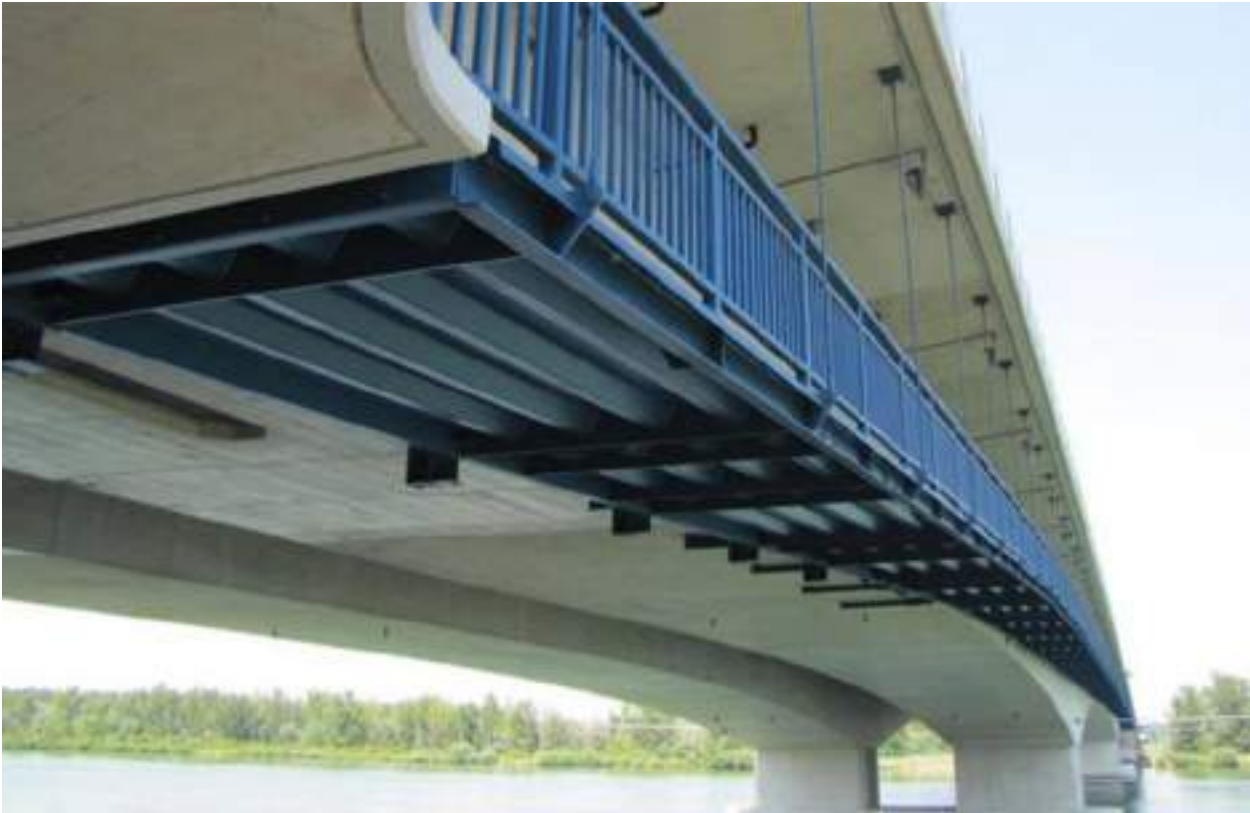
Figure 44. Cycle track on the lower level of the S33 expressway bridge across Danube, Austria.
