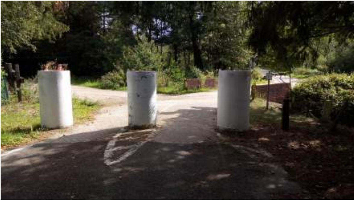
Figure 6. Typical bollards are prone to vandalism in remote rural areas, so more sturdy constructions are sometimes used to prevent unauthorised passage.
