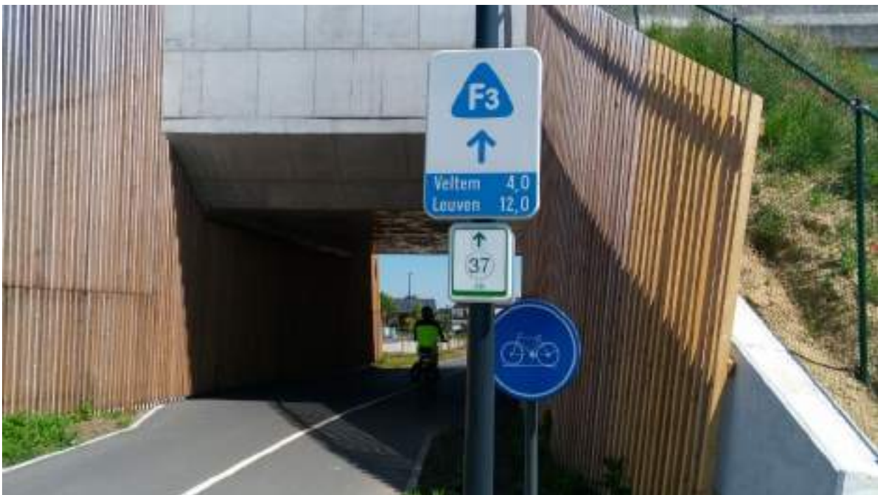
Figure 24. The cycle path and tunnel is a part both of the F3 cycle highway (upper sign) and the node network (lower sign, directing towards node 37).
