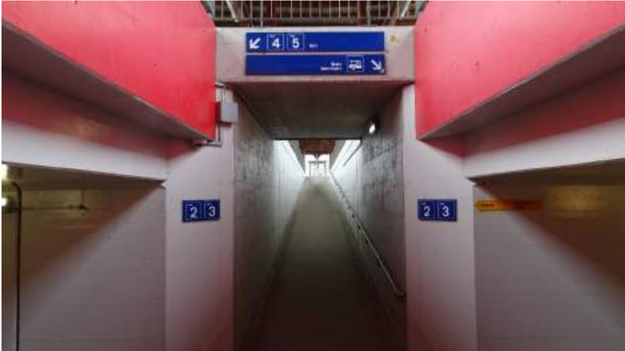
Figure 47. Simple, straight ramps provide a more reliable and higher capacity access to platforms than lifts. Stein-Säckingen, Switzerland.
