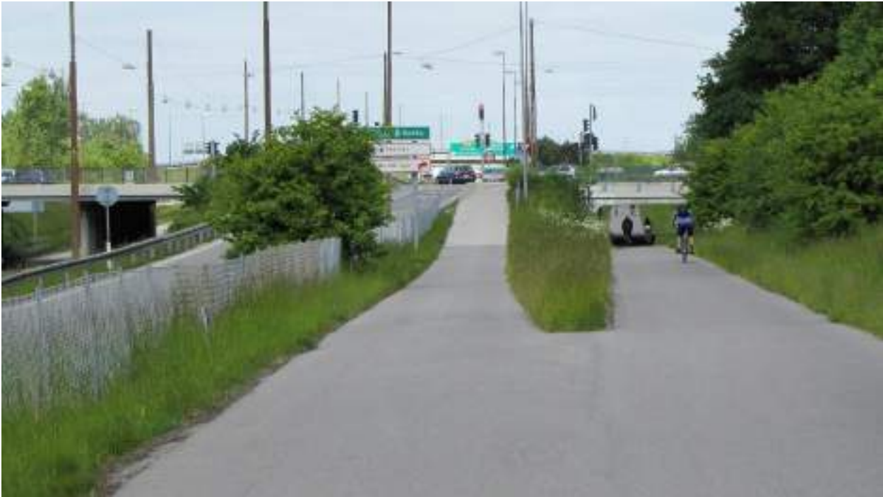
Figure 42. Cycle tracks along a motorway integrated in the interchange design. Farum Route, Greater Copenhagen.
