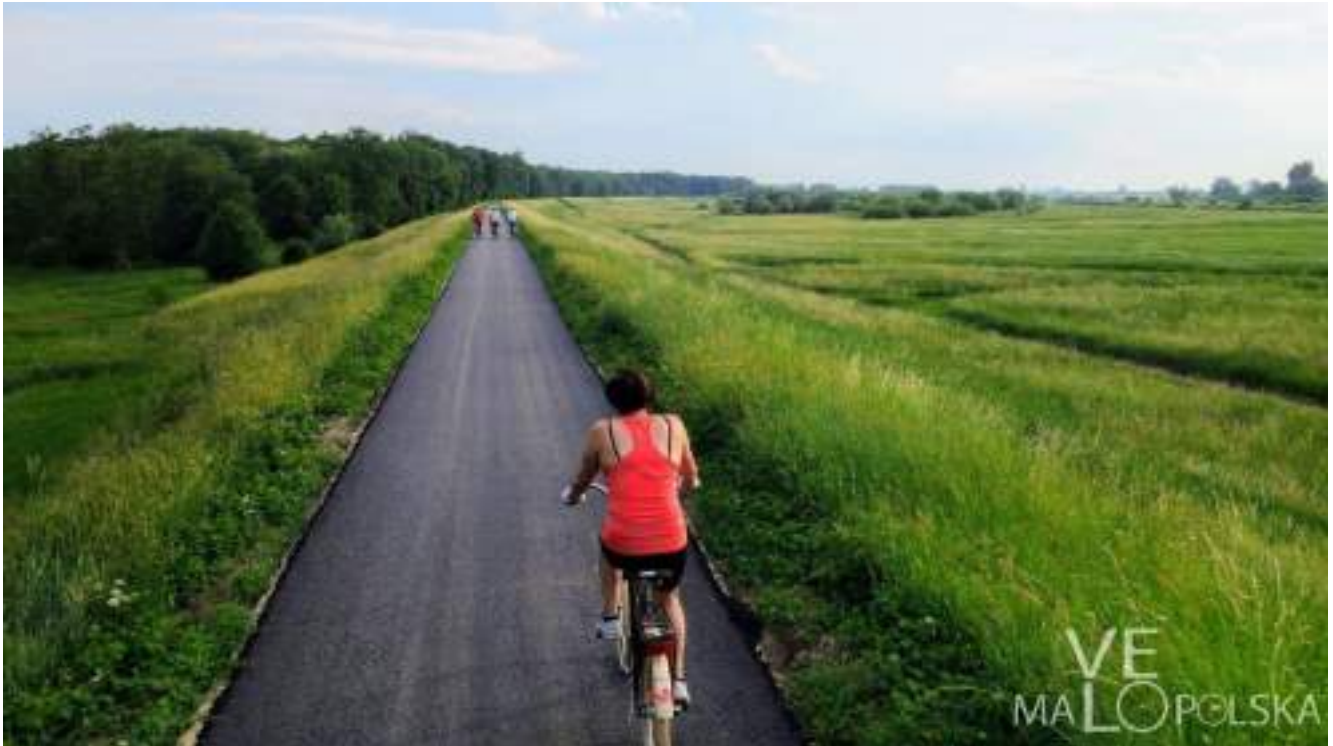
Figure 51. Cycle track on a levee in Malopolska, Poland. Photo credit: VeloMalopolska.
