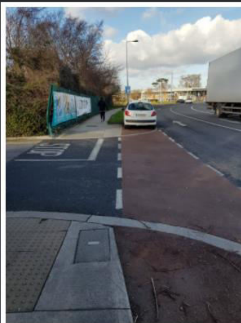
Whole lane blocked, job done!
